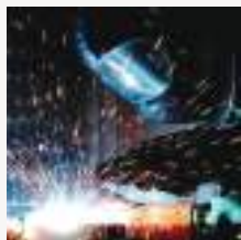
Welding fumes suction
